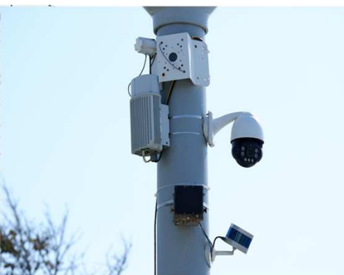
Smart Lamp Post (ITS-G5, C-V2X, 5G, Wi-Fi, LoRa)+mmWave+ sensors
